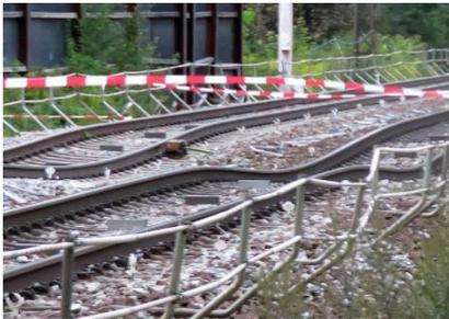
Earlier this week the already grim situation got suddenly worse, when tunnel construction in the town of Rastatt resulted in unexpected damage to the double track Rhine Valley mainline. The tunnel boring machine that was crossing a few metres below the railway line caused a serious deformation of the tracks, making them unsuited for traffic.
